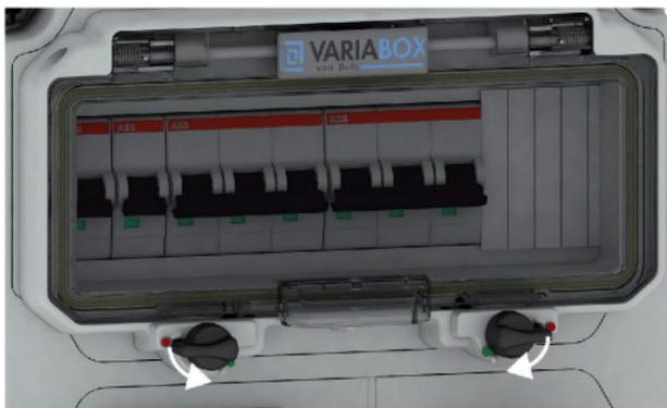
4. Open the OTC flap completely. In doing so, overcome the perceptible resistance until the flap latches audibly in the completely opened position.
